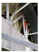
The scaffold utilises 5km of tubing, 12,000 fittings and 500 timber boards, every piece of which has to be lifted into place by hand.
