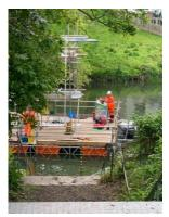
Before any structural repairs can begin, a scaffold has to be erected below the bridge to create a working platform. A floating pontoon was assembled in the river, from which the scaffold can be lifted. This also enables us to keep the bridge in use for traffic under controls.
