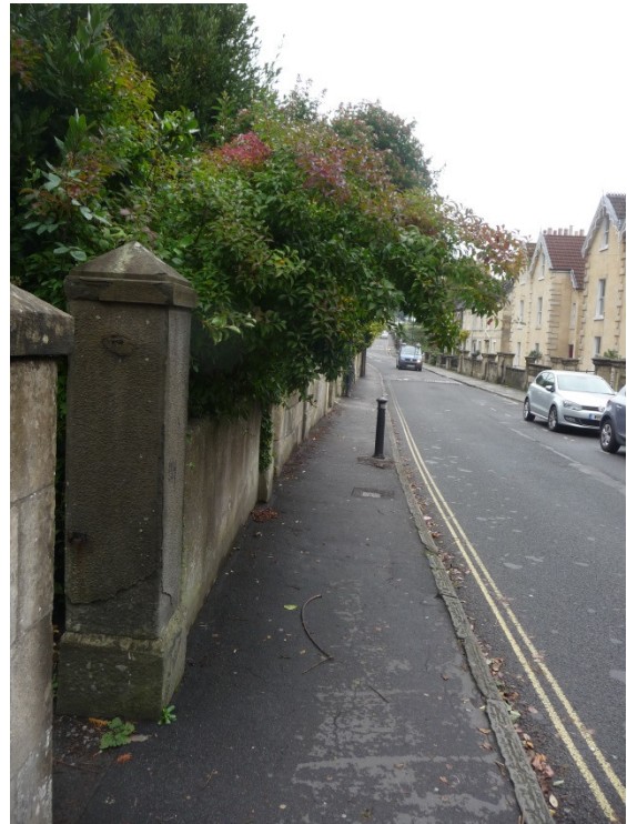
Vegetation overhanging the narrow pavement in Camden Road
